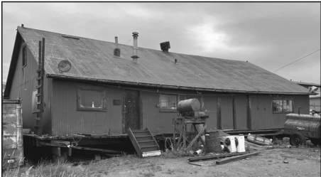
Structure 2 – Shop Building (approximately 58’ x 39’)
